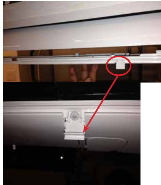
Figure 58: Remove Screws from Bottom Panel
