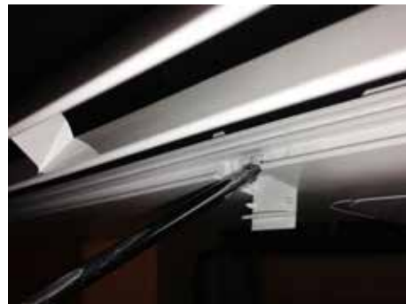
Figure 59: Remove (and Reattachment) Bottom Panel
