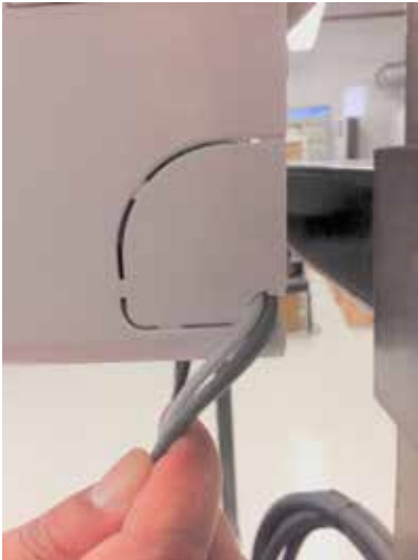
Figure 60: Indoor Unit Knockout (Communication Wires)
