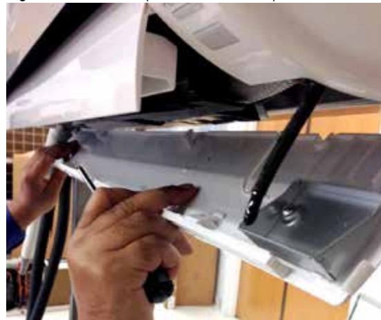
Figure 59: Remove (and Reattachment) Bottom Panel
