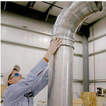
Lift pieces into place
