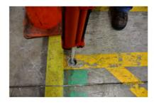
Insert the SFD gauge into the hole. It is critical to STOP the adhesive at contact with the gauge to ensure you do not over fill the opening.
