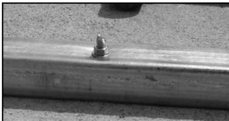
4. Repeat for each anchor bolt until base rail or rails are adequately secured to the concrete base.
