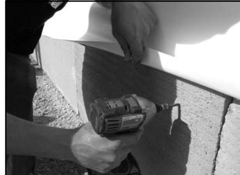
**NOTE:** Hole needs to be deep enough that the anchor bolt will not interfere with ratchet operation.
