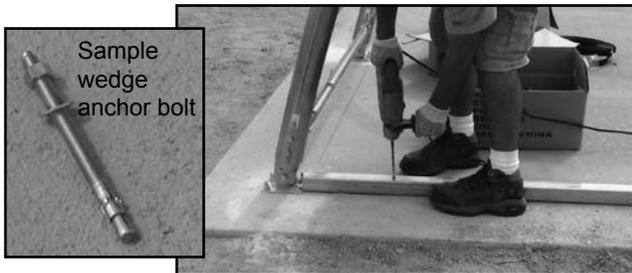
**IMPORTANT:** DO NOT over-drill hole. Wedge anchor bolt will not work properly if hole is too deep.
