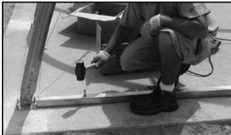
**NOTE:** Depending on wedge anchor bolt, verify that the washer and securing nut are attached *before* driving the anchor bolt into concrete. Striking bolt may cause thread damage and prevent the nut installation.
