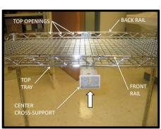
STEP 7 – USING TWO (2) 3/8" X 1" LONG BOLTS, FOUR (4) FLAT WASHERS, TWO (2) LOCK WASHERS, AND TWO (2) NUTS, ATTACH THE CENTER CROSS SUPPORT TO THE TOP SHELF. TIP: USE THE SIXTH TOP OPENING IN THE FRONT/BACK RAILS OF THE TOP SHELF.
