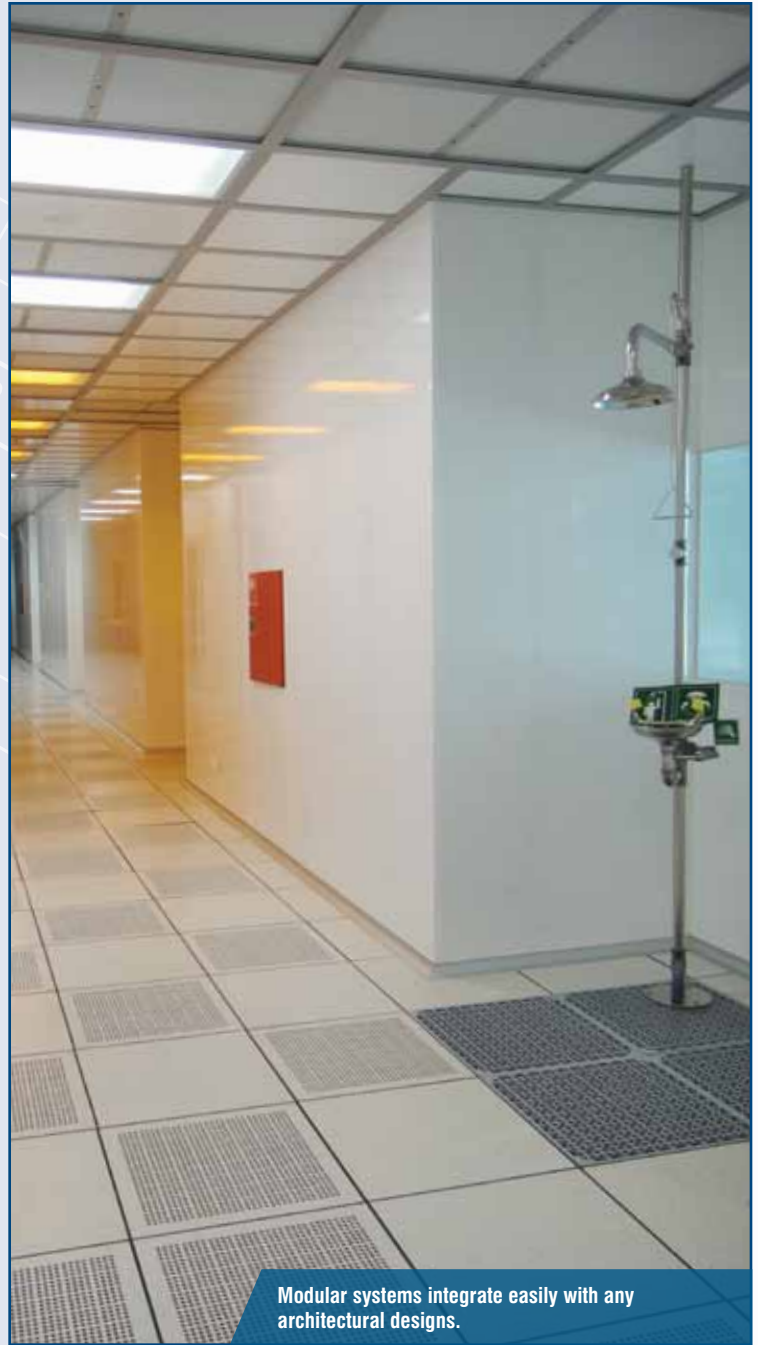
Load-bearing plenum decks provide a maintenance platform eliminating the need for a separate catwalk.
