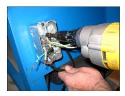
Step 9: Connect wires per schematic. Connect all three ground wires and attach mechanically to box per code. Wire nut all connections.
