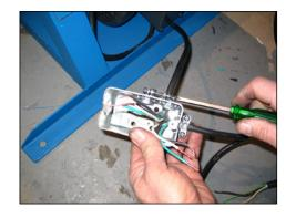
Step 7: Install safety switch wire through the middle side hole. Tighten screws.
