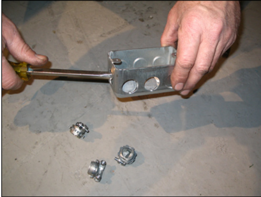
Step 1: Remove 4 knock outs from provided junction box.
