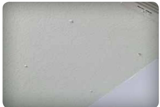
3. From below, place the cut-out template on the ceiling at each location, making sure that you have at least 2 inches of clearance all around it. While holding the template in place, mark its outline with a pencil.
