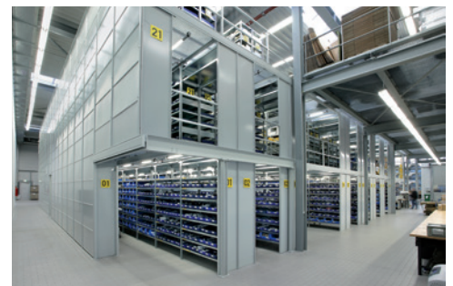
3-tier storage facility in the automotive industry.
