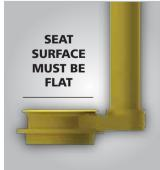
**Step 11**: Check for flat surface on seat. Any damage to seat will require replacement of the entire brass seat with Fluidmaster's 507 Flush Valve.
