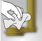
**Step 12**: Wipe down the BRASS FLUSH VALVE SEAT before installing to check for mineral build-up. If the OVERFLOW PIPE is threaded on (some are, some aren't) make sure it's tight by twisting clockwise before installing the BRASS SEAT ADAPTER.
