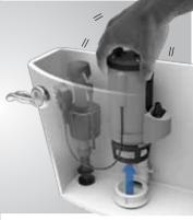
Once released clean seat and inspect piston seal at bottom ensuring the seal is centered oh piston. Reattach DUO FLUSH<sup>™</sup> and handle actuator. Turn on water and recheck water level for leaking.
