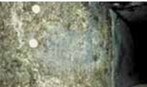
Result w/ Fibrous: Mold growth on insulation
