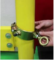
**6.** Measure each bollard ring from the floor to set height of the opposite 4 rings that will be installed next. Now that you know your heights measure, mark the placement, and finally slide the ring to place and repeat steps for securing your safety ring.
